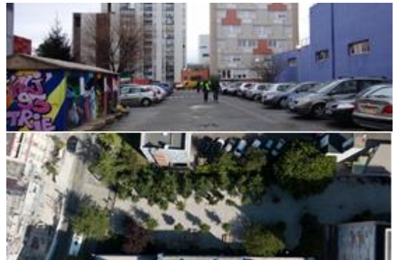
Figure 11 : Parking AVANT/APRES la transformation - © Fieldwork Architecture
